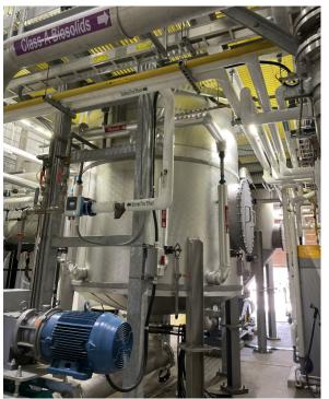
This advanced biosolids management project includes the implementation of a Lystek THP LY10 Module alongside a dewatering centrifuge and permanent biosolids truck loading infrastructure. The project took advantage of existing liquid storage tanks and building infrastructure to optimize the use of existing infrastructure and minimize capital costs.
