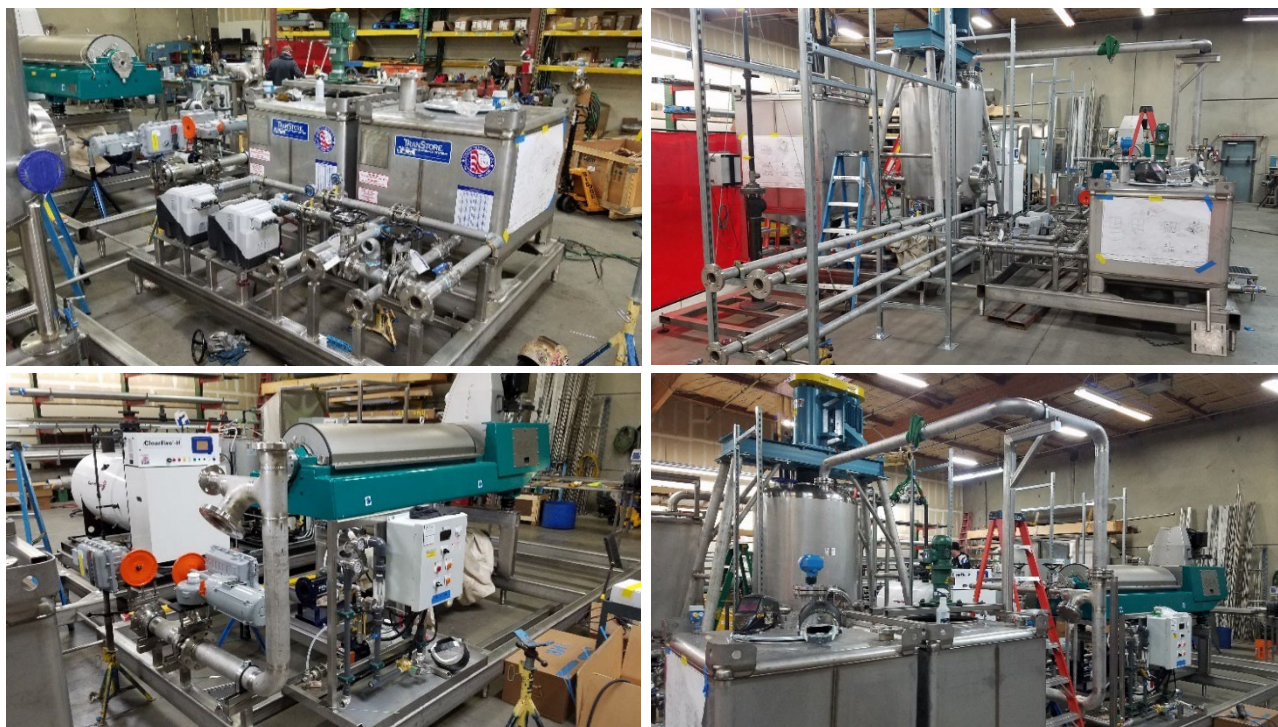
Figure A-1: Shop Fabrication of the Process Skids
