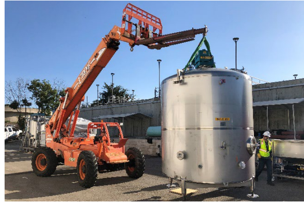
Figure A-2: Installation of the Skids at Goleta Sanitary District
