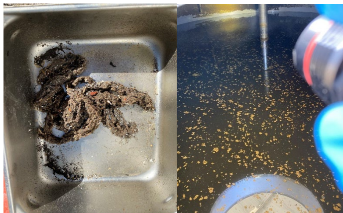
Figure 25: Solids Observed during Digester Cleanout
